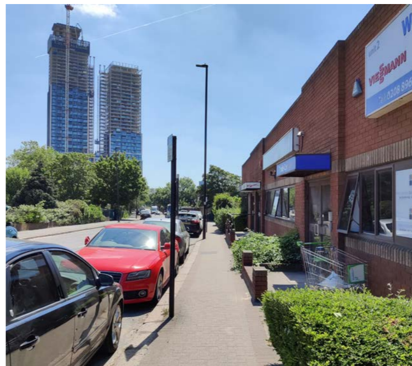
3. View from Park Royal Road looking south
